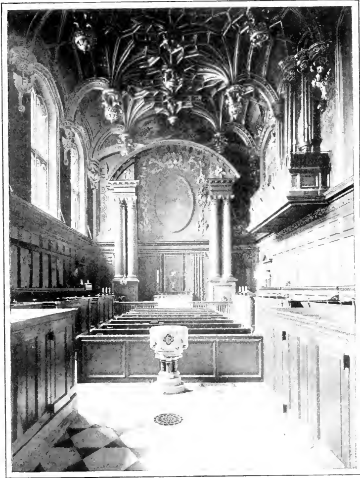
THE CHAPEL, HAMPTON COURT PALACE.
